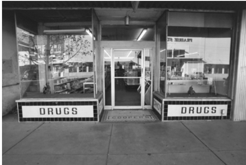
Photo 7: Ceramic tile storefront bulkhead and entry. Note deeper recess and entrance and stairway to upper floor on left.
