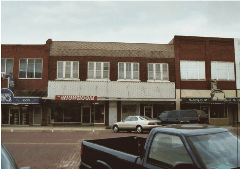
Photo 1: View of building exhibiting horizontal orientation. Note metal transom cover to be removed.
