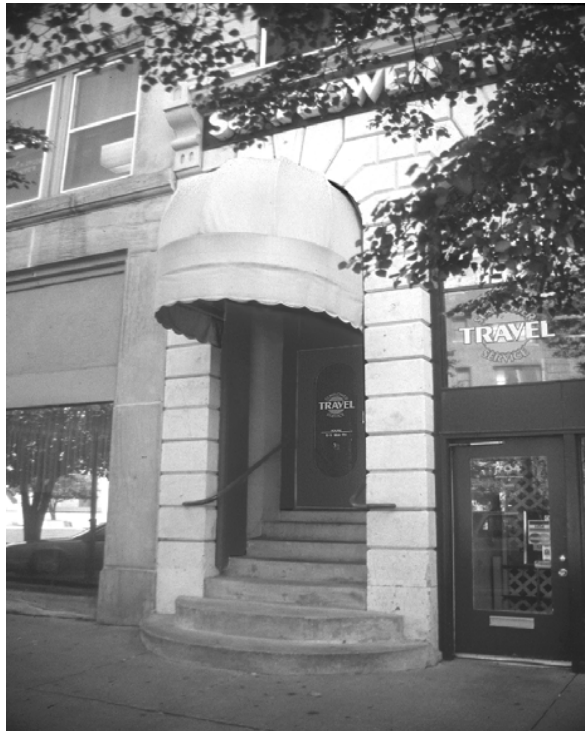
Photo 6: Example of a simple awning over an entrance providing emphasis and weather protection.
