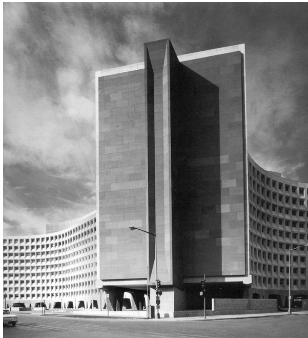
Photo 4: Example of Expressionism. U.S. Department of Housing and Urban Development Building.
