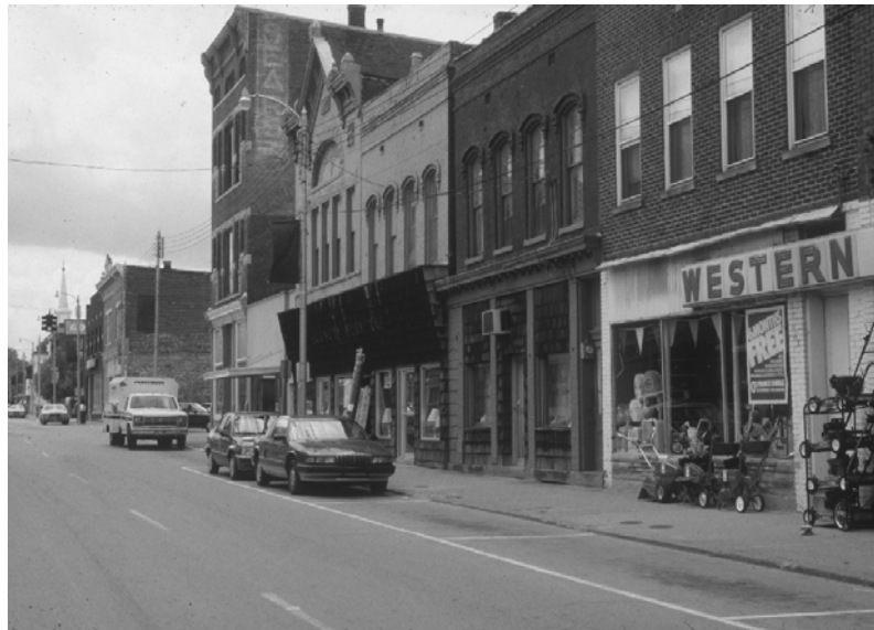
Photo 1: An example of inappropriate first floor “modernizing” of facades on buildings dating prior to 1920.
