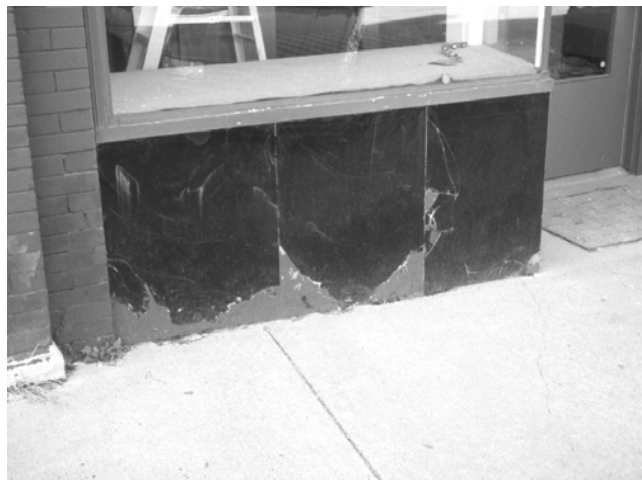
Photo 3: Example of original storefront bulkhead replacement c. 1930's using pigmented structural glass, which is currently in need of repair or replacement.
