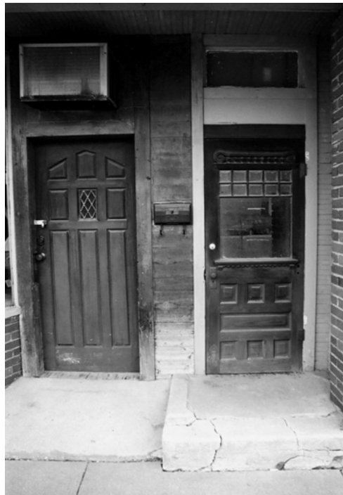
Photo 2: Example of step-up at building entry that limits access.
