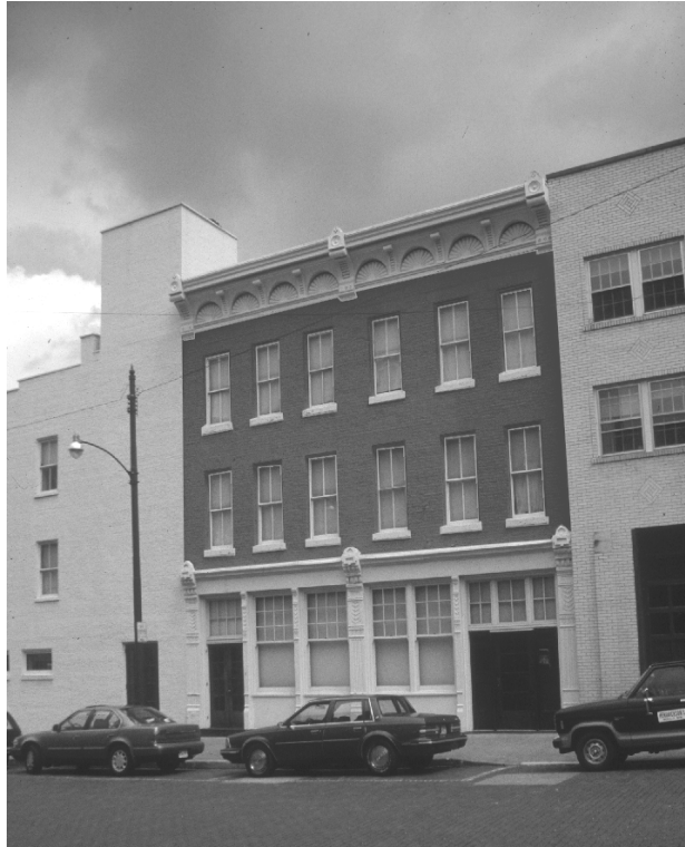
Photo 7: Example of a pre 1920 building in a solid light color on metal work with darker accents at doors. Note decorative pressed metal cornice is painted a solid color.
