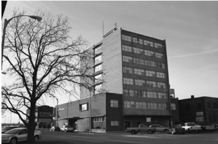
Photo 1: Example of early 1950's International Style building. Note expansive glass areas, straight linear lines, and cantilevered planes over entrances.
