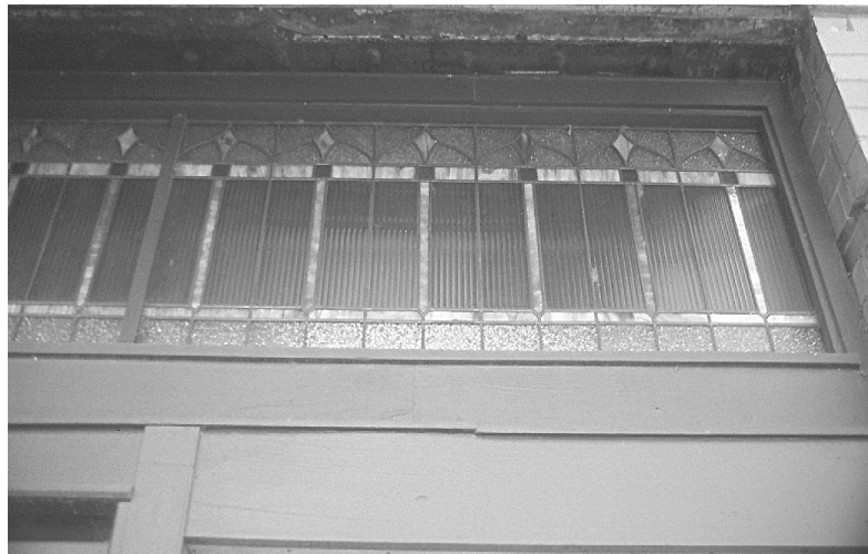
Photo 5: Example of ornate glass transom window that allowed light to penetrate deeper into the space than lower windows would allow.
