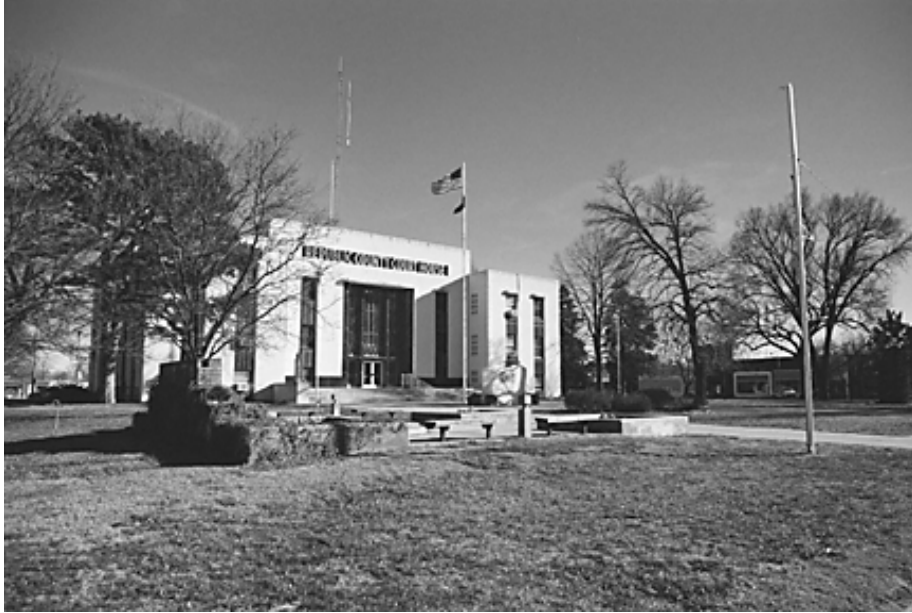
Photo 3: View of the Republic County Courthouse, looking east. A Historic Register listed building which is an excellent example of the Art Deco architectural style.
