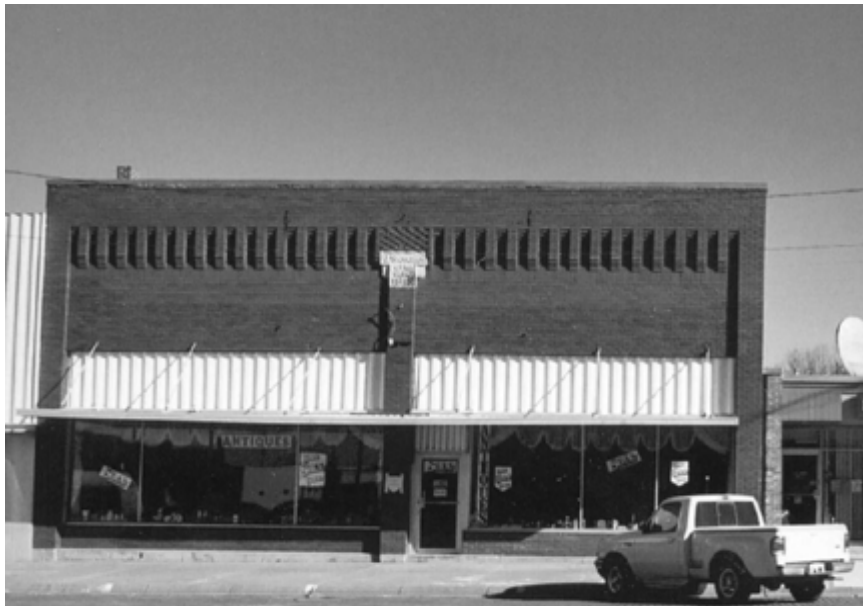
Photo 6: An example of a corbeled brick cornice.
