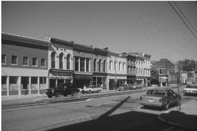
Photo 2: A series of downtown buildings exhibiting regulating lines. Note the alignment of upper and lower cornices, transom windows, window heads, etc.
