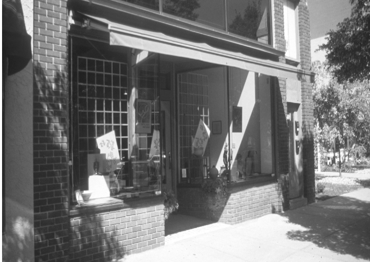
Photo 4: Example of a well designed, well lit display window illustrating good merchandising techniques. The building is clean and well maintained. Note roll up awning and mailboxes at side door indicating living spaces available on upper floor in downtown area.
